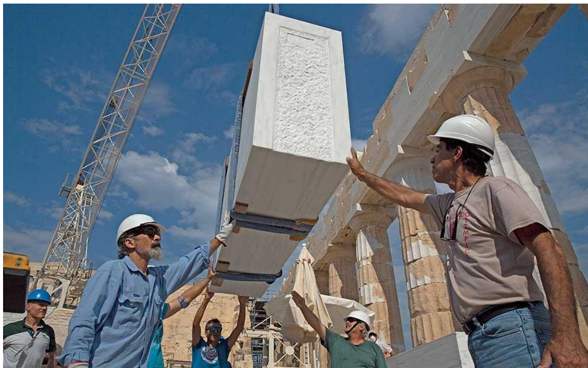
After placement, the addition's upper surface receives treatment so that the next block or blocks will sit correctly on top of it. © Nikos Pilos
