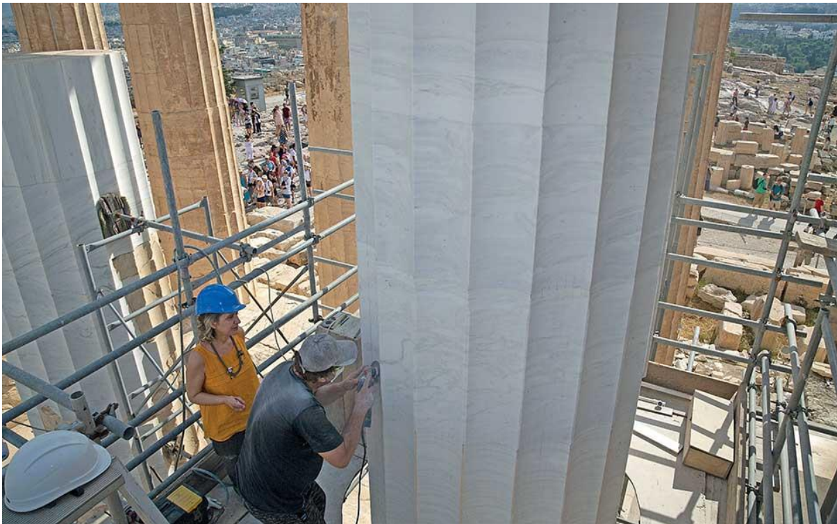
Highly experienced marble masons work on site as they carve the flutes of new drums set in the pronaos columns, using both modern and traditional tools. © Nikos Pilos
