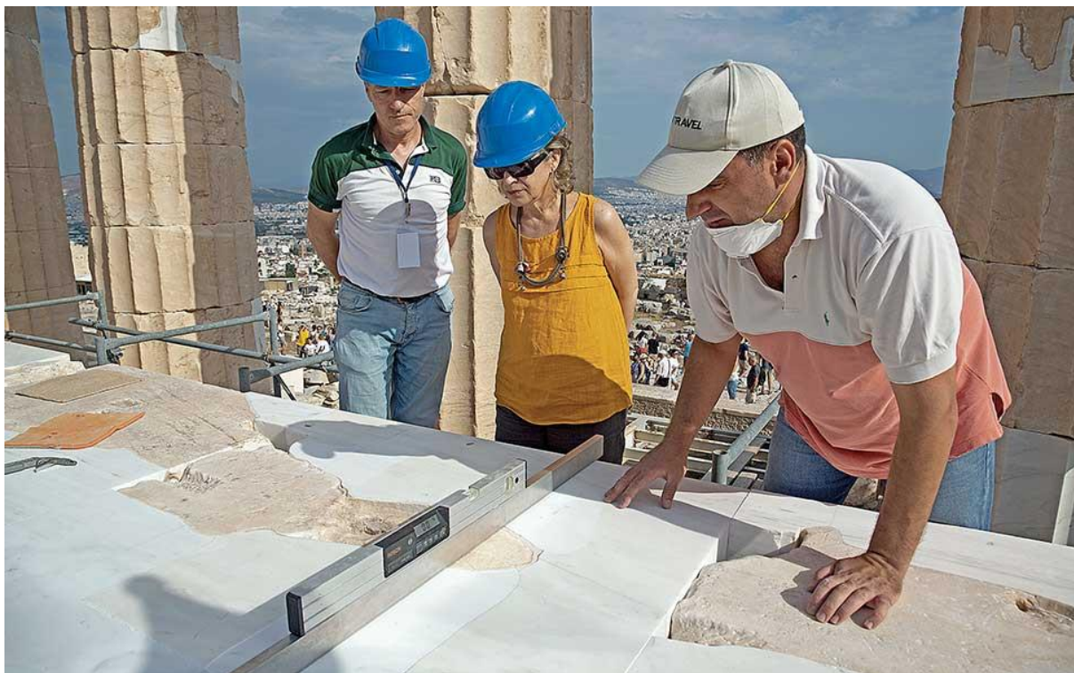
Tentative placement of an orthostate block, created from new marble, weighing 4 tons.
